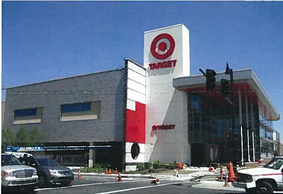
The Target store on Penn Avenue in East Liberty, days before its opening July 24, 2011.
